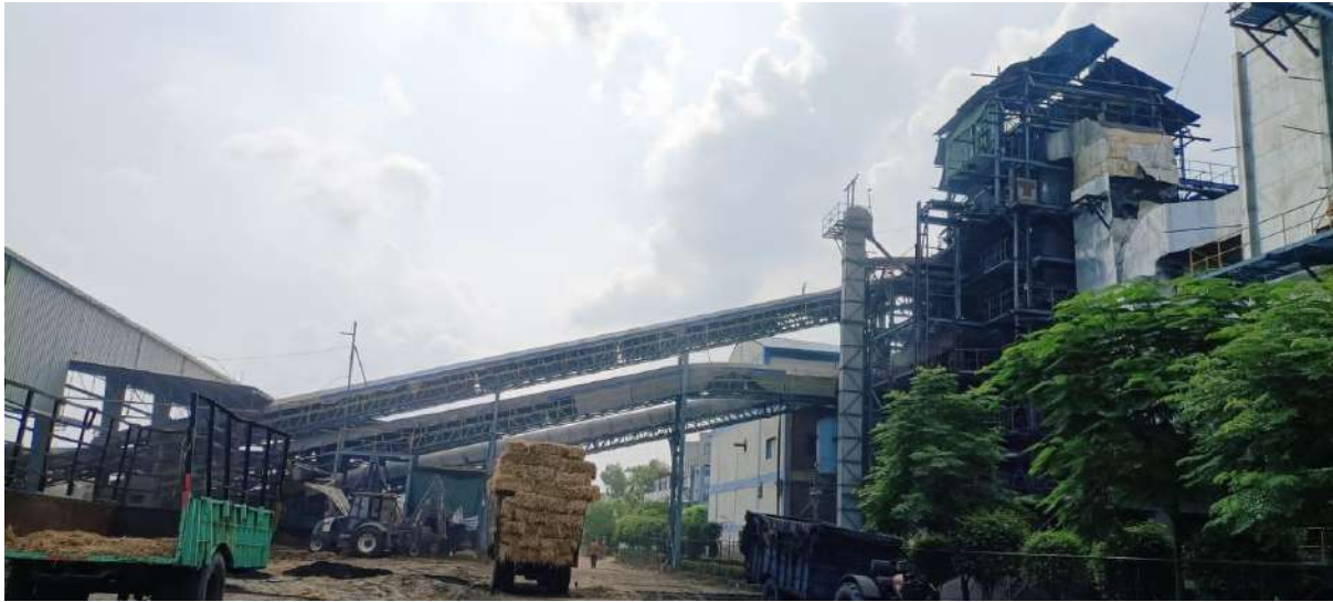
Biomass Power Generation Facility 1- DEE Power Operated under DEE Development Engineers Limited (Holding Co.)
